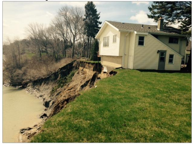
Figure 3.7.2-1: Bluff failure in Mount Pleasant, 2016.
