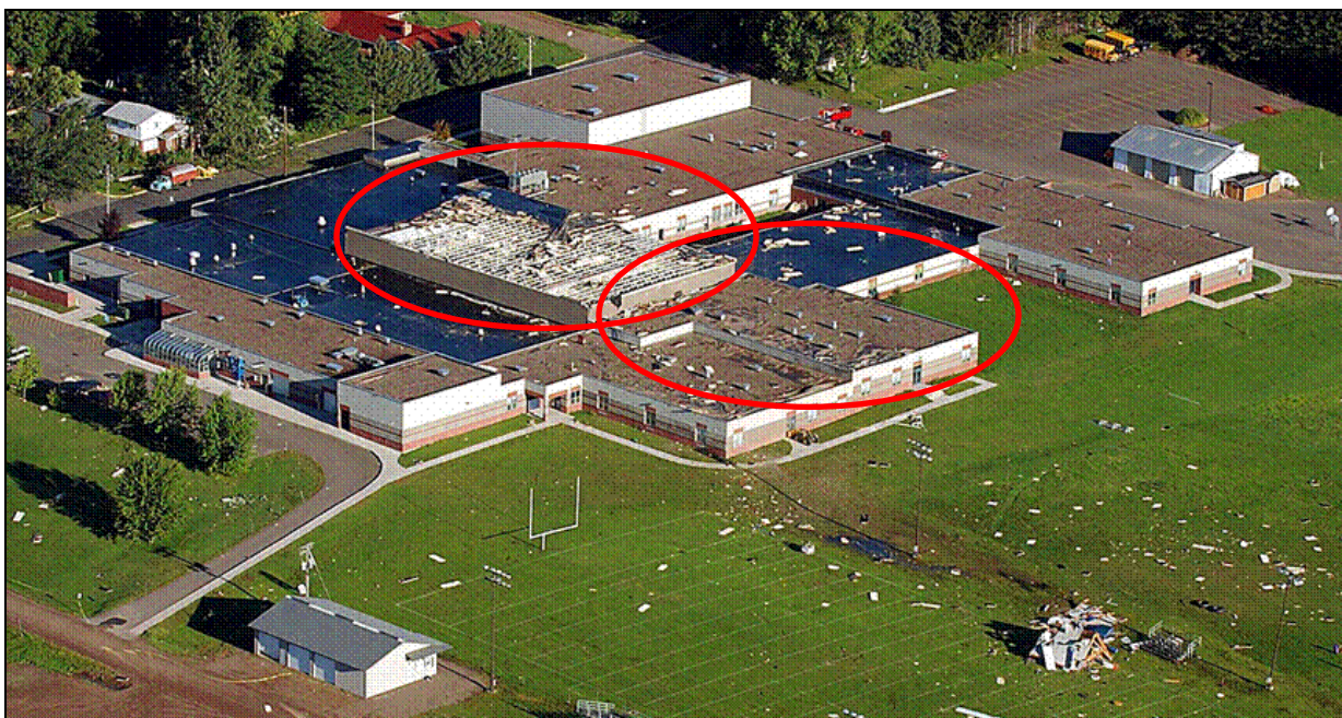
Figure S-1. Damage to the Gilman School. Damaged gymnasium and classrooms are circled (Photo by the Eau Claire Leader-Telegram).
