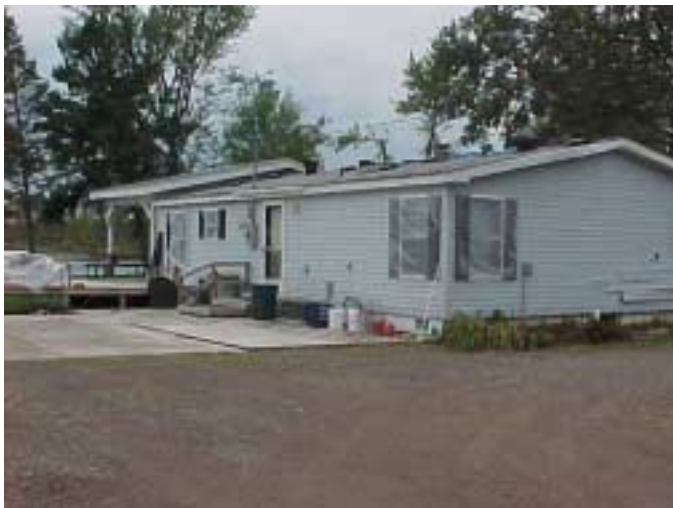
Figure R-15. Windows damaged and covered with plastic (700 River Street, Ladysmith)
