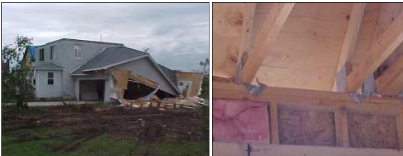
Figure R-12 and R-13. Loss of garage door allowed wind inside garage. Roof trusses in garage moved from original position. Nails were used to secure clip to wall top plate, but no nails connected the clips to the trusses (607 Lake Avenue, Ladysmith).
