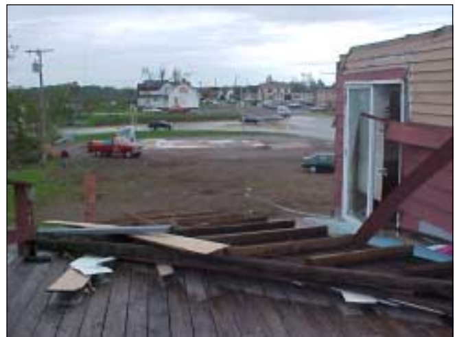
Figure R-8. Gable end wall was pulled off of building. (Lake Avenue, Ladysmith)
