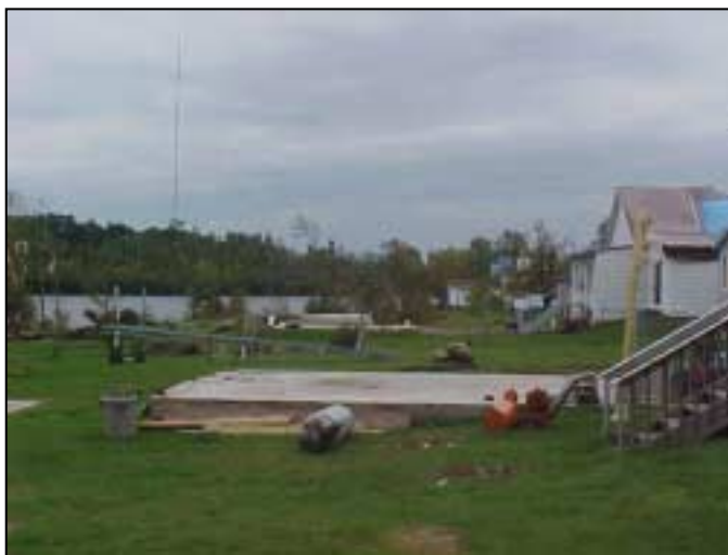
Figure R-14. Storage sheds and garages destroyed due to poor anchorage to foundations. (Residences along Lake Avenue, Ladysmith)
